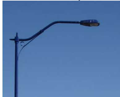
Summerside Area 70 Street SW – Stanton Drive SW South of Ellerslie Road
